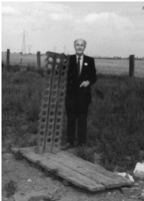
Bill Hunt visited the Foggia airfields in 1992, finding a section of PSP (Pierced Steel Planking), which made possible the building of improvised runways.
